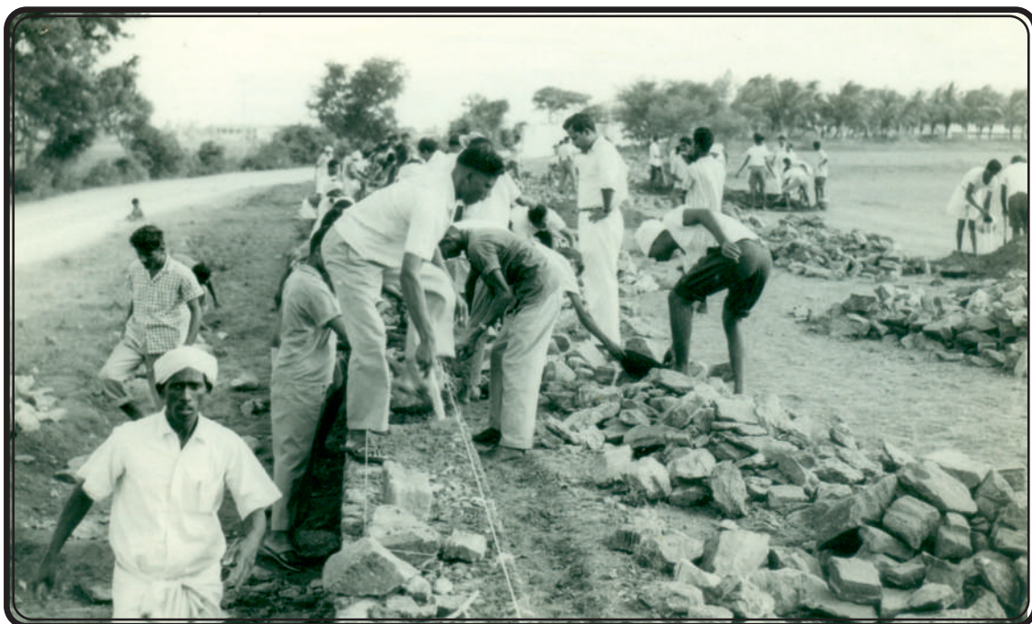
Compound Wall Construction
